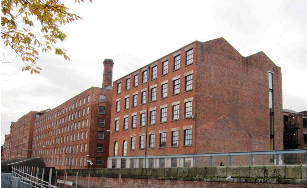
Figure 2: Royal and Murrays' Mills by the Rochdale Canal.
