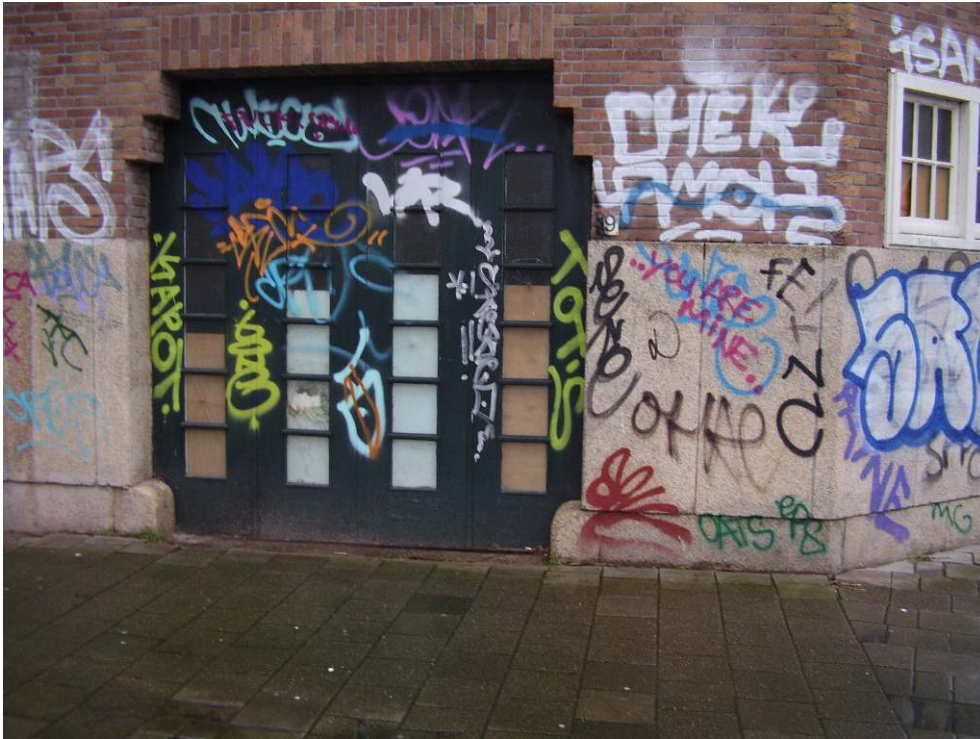
Figure 3. Disrespecting the unwritten rules of graffiti: writer's crossing each other's tags out.
