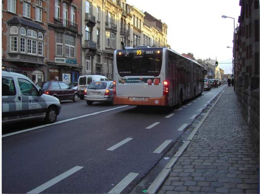
Figure 10: Bus lane that disappears as it approaches a crossroads (Avenue de la Couronne/Kroonlaan, a regional thoroughfare)
