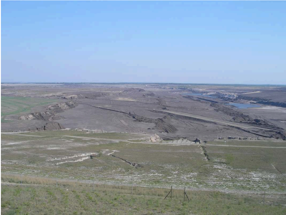
Photo 1. Residual cavity of the Meuro mine in Großräschen (Deshaies, 2007). Closed in 1999, the flooding of the Meuro mine began in 2007 to form Lake Großräschen.
