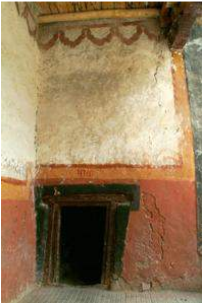
Fig. 6. Doorway to the Mangyu eastern tower
