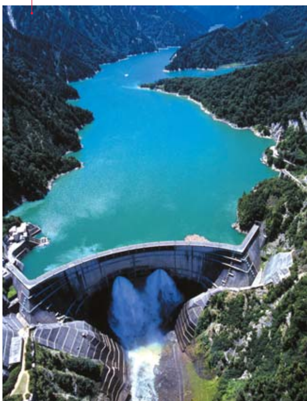
Kurobe Dam, in Japan, is designed mainly to combat flooding (photo: ICOLD-CIGB)
