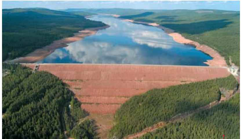
The Trångslet Dam in Sweden (photo: ICOLD)
