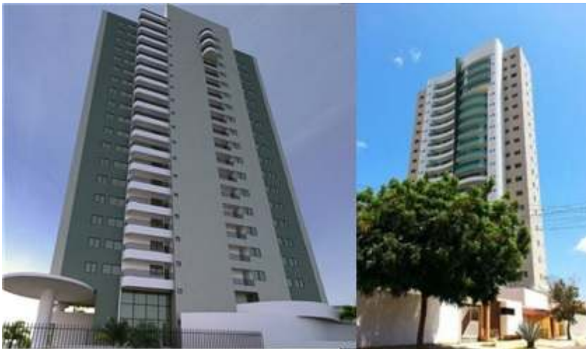
FIGURA 6 -Condomínio Splendore Residence
