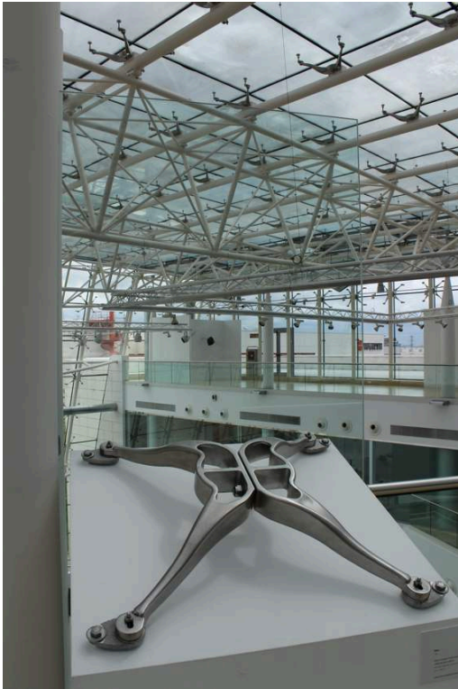
Fig. 6 – Agoncillo. Museo Würth, Agoncillo. Garra (staples anchoring the glass cover), exhibited in the museum as a sculptural work.
